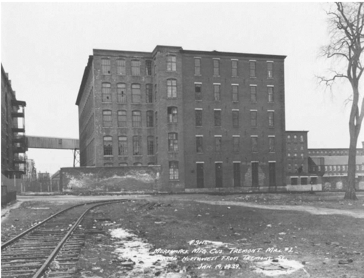
Tremont Mills Powerhouse and Mill No. 2 as seen in 1939. (Photo – Lowell National Historical Park)
