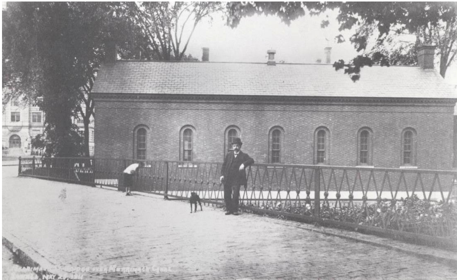
View of the Moody Street Feeder Gatehouse on Merrimack Street in 1911. (Photo – Umass Lowell Center for Lowell History)
