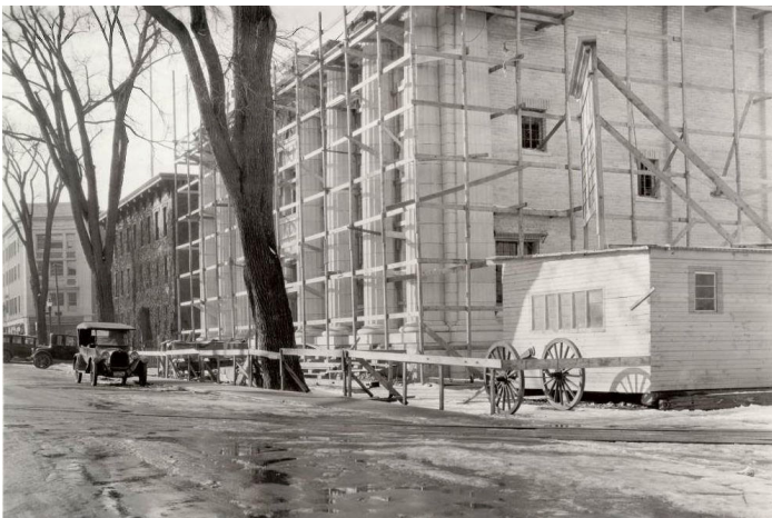
View of the Masonic Temple under construction on December 14, 1928, looking toward Merrimack Street. (Photo – Lowell National Historical Park)
