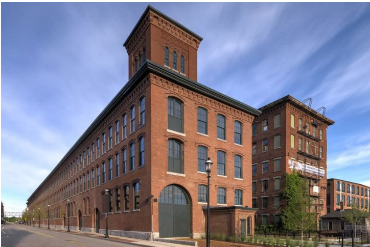
Counting House Lofts on Jackson Street.
